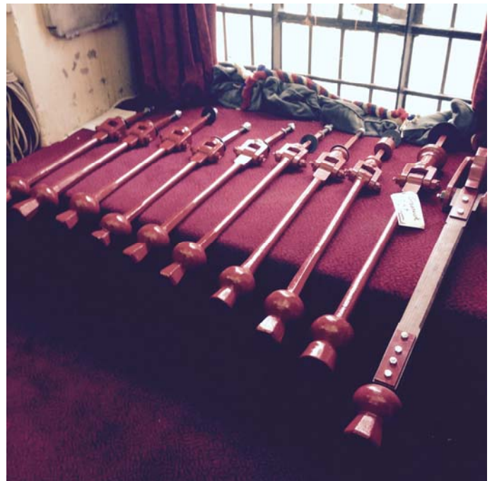
The clappers, including the new wooden shafted tenor clapper, on the ringing chamber floor prior to being reinstalled.
